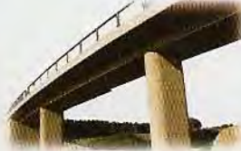
a concrete bridge
